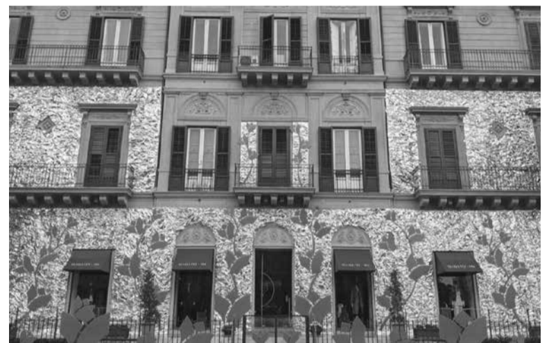
Giglio's shimmering new façade
